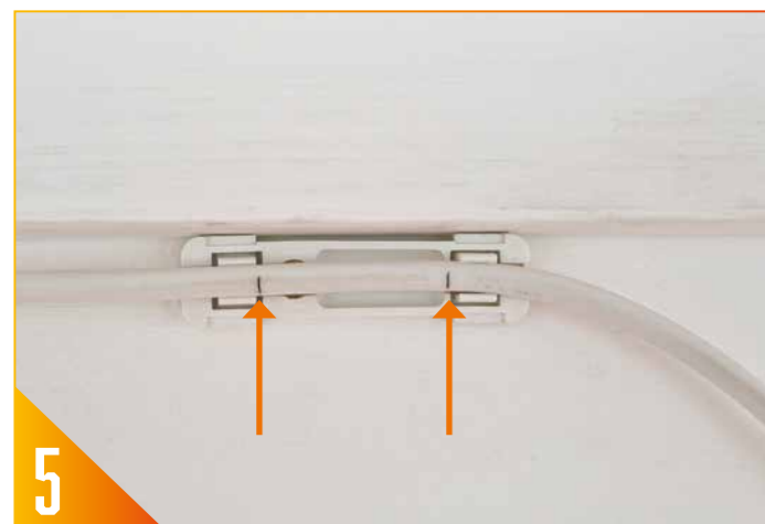
5 Place the cable within the Break-Out Bend Manager and mark start and end points for a window cut.
