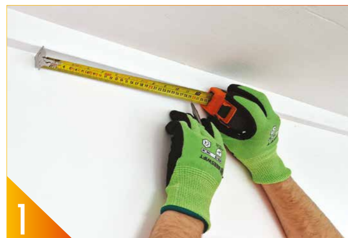
1 Mark out 300mm lengths between each required FireClip.
