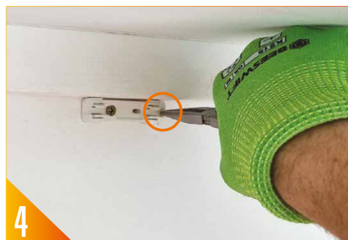
4 Place and fix to the wall with a screw and if the cable is continuing its route for more fibre drops, remove the end cap to allow the cable to pass through.
