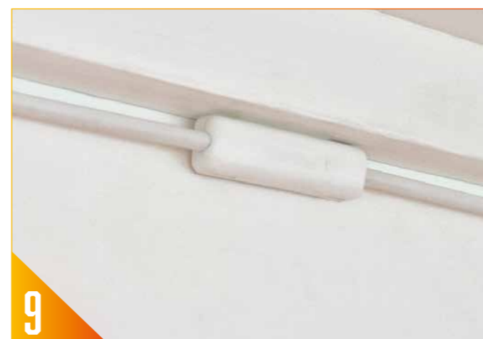
9 When complete, push on the cover for the Break-Out Bend Manager until it clicks into place.
